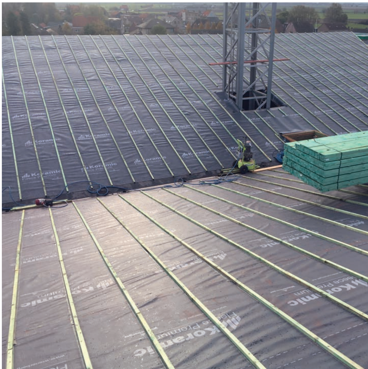
Fleece Premium + Nail-Tape Butyl nageldichtingsband
